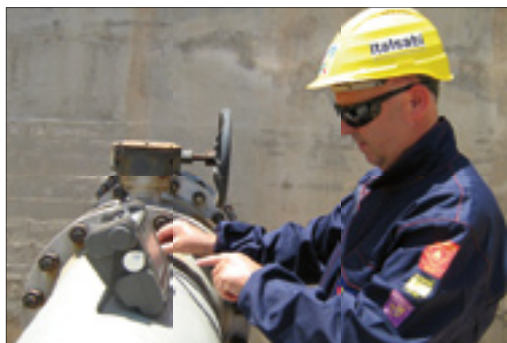
▲ Critical defect examination with ultrasounds
